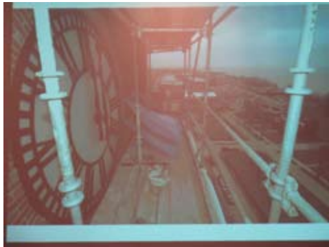
Great Lakes Building 1 Clock Restoration Photo
